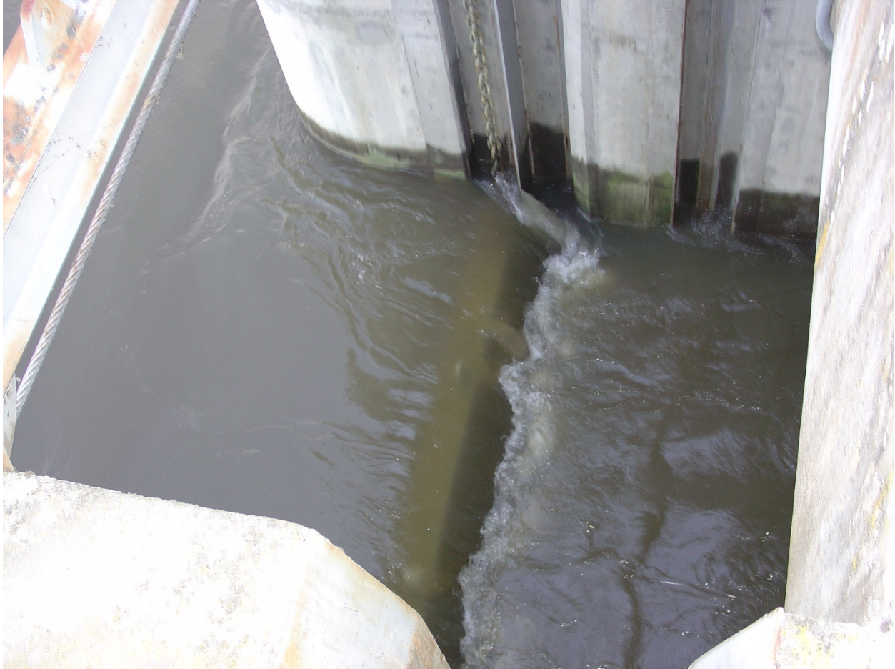
Figure 3. Tailrace overtopping closed fishway entrance SSE2 at Ice Harbor Dam.
