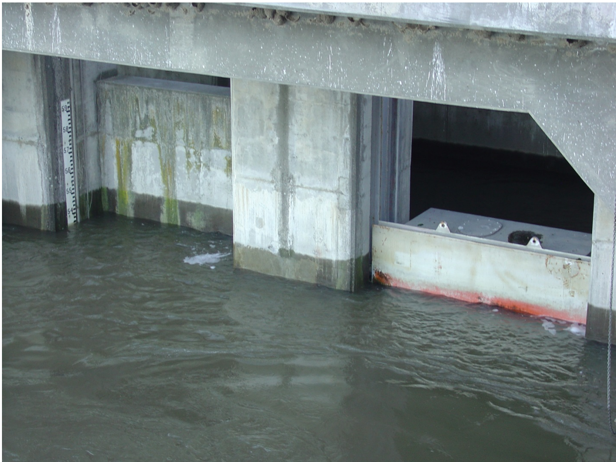
Figure 1. IHR operating floating orifice, sometimes referred to as a FOG (floating orifice gate).
