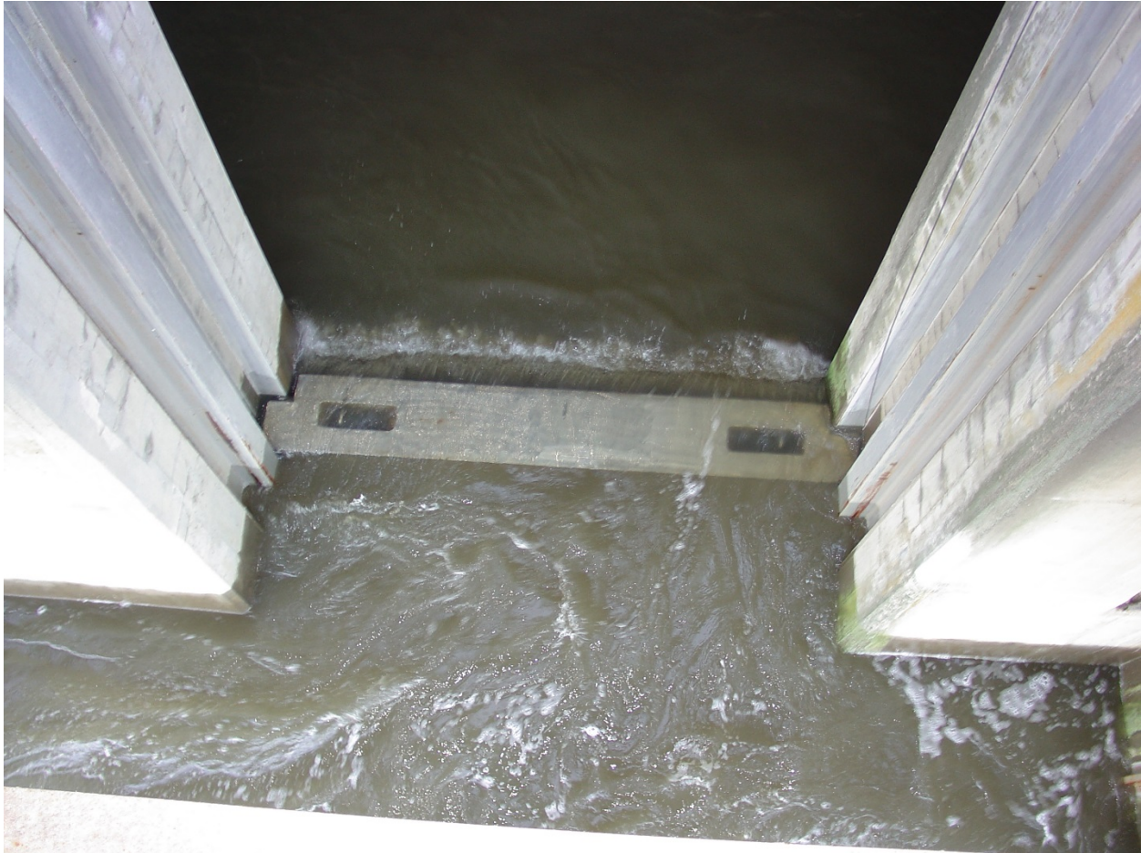
Figure 2. Tailrace overtopping closed floating orifice at Ice Harbor Dam.
